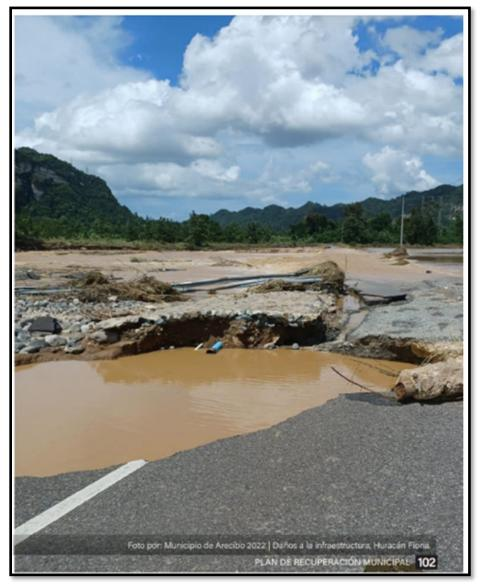
Figure 27: Road Damage near Jurutungo sector and the Río Grande river in the Municipality of Arecibo. MRP Plan Municipality of Arecibo.
